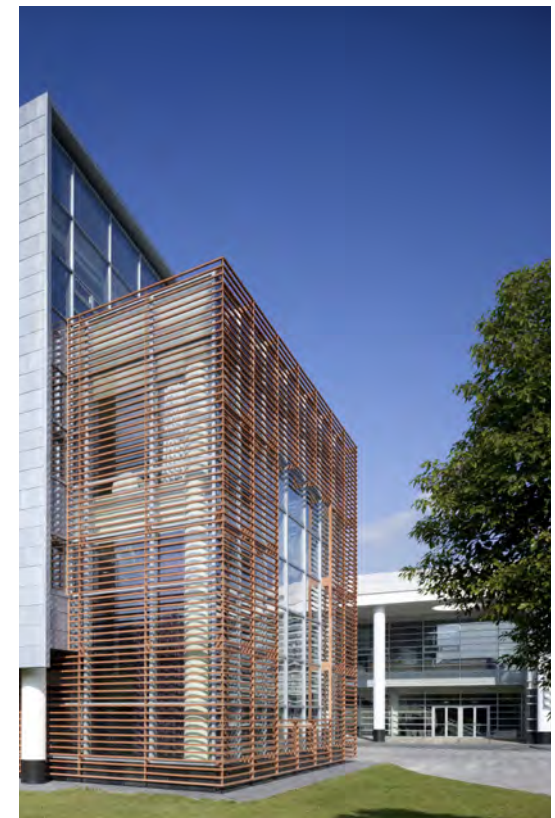
Concordia International School | Elementary School Photo courtesy of Perkins Eastman | Photographer: Tim Griffith
